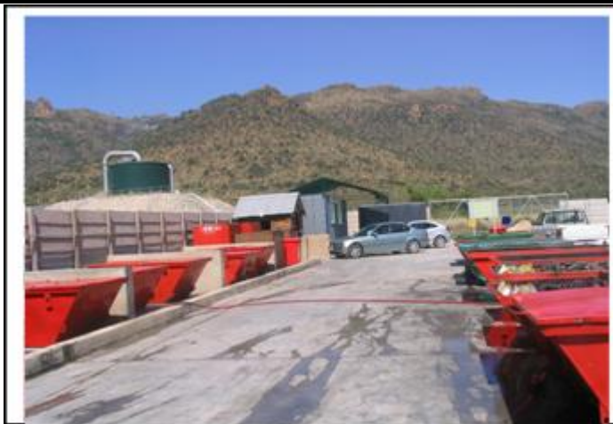
Figure 1.3 Oily Waste Management Facility
